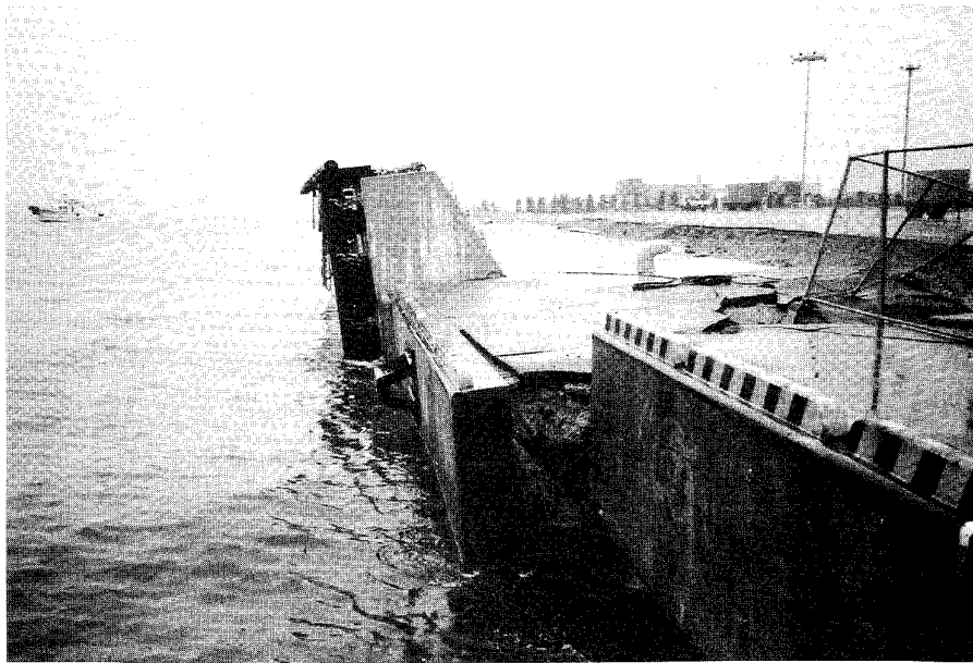
Figure 1.14 Failure of a quay wall on Rokko Island in Kobe, Japan in the 1995 Hyogo-Ken Nanbu earthquake (photo by S. L. Kramer).
