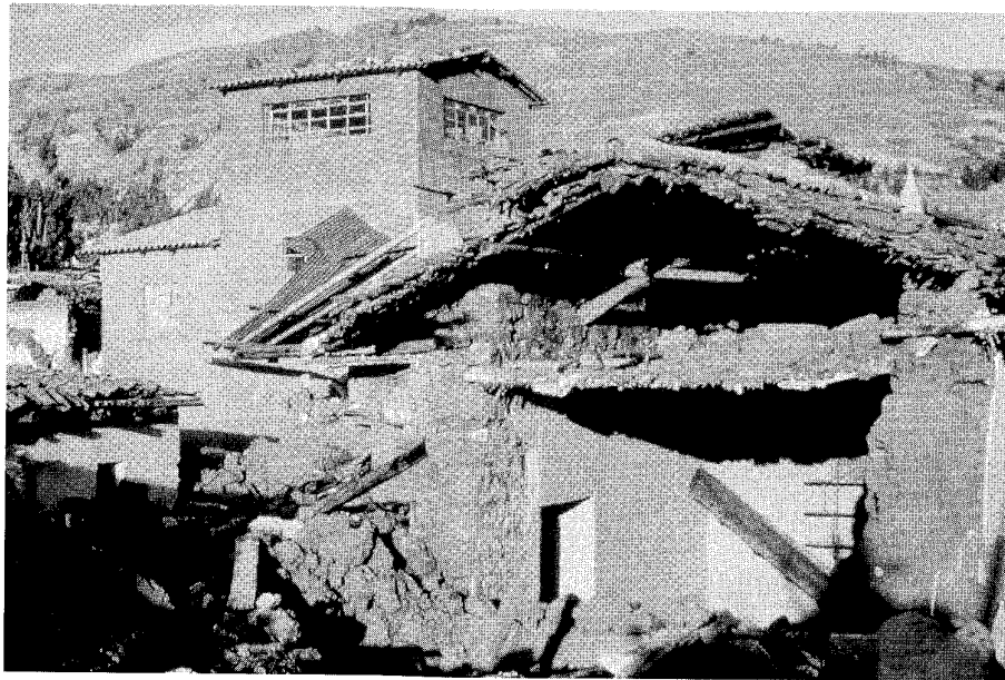
Figure 1.1 Damage to buildings in Huaras, Peru following the 1970 Peru earthquake. The adobe structures in the foreground were destroyed, but the reinforced concrete structure in the background suffered little damage (photo by G. Plafker, courtesy of USGS).
