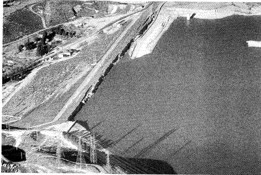
Figure 1.7 Lower San Fernando Dam following liquefaction failure of its upstream slope in the 1971 San Fernando earthquake (K. Steinbrugge collection; courtesy of EERC, Univ. of California).
