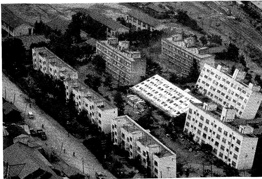
Figure 1.6 Liquefaction-induced bearing capacity failures of the Kawagishi-cho apartment buildings following the 1964 Niigata earthquake (courtesy of USGS).
