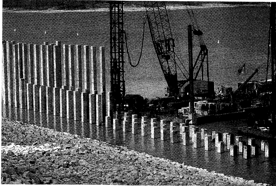
Figure 12.8 Compaction piles driven into the upstream embankment of Sardis Dam to reduce liquefaction hazards. The contractor drove the piles to this level with a barge-mounted conventional hammer; the piles were later driven below the water surface with a different hammer. (Photo by T. D. Stark; used with permission.)
